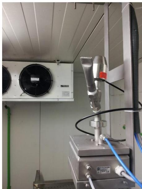
Picture 3: Fogging unit in cooling room
